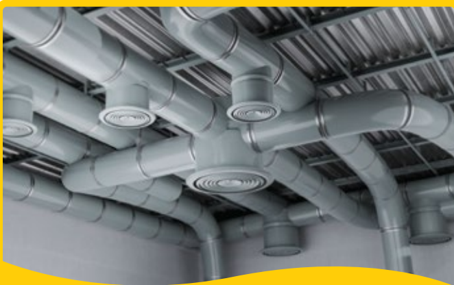
FABRICATION & ERECTION OF PIPE SPOOLS
