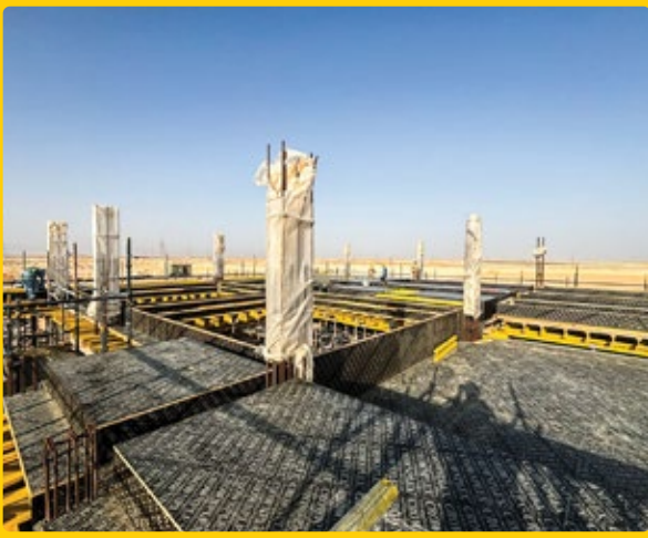
8. CONSTRUCTION OF CONTROL STATION BUILDING FOR STS PDO AT AMAL
