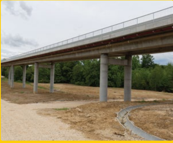
1. CONSTRUCTION PDO FIELD ACCESS ROADS
