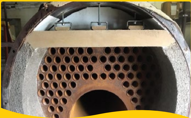
OTSG/HEAT EXCHANGER – REFRACTORY REPAIR WORKS
