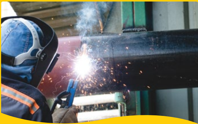
WELDING OF PIPES (ARGON & ARC)
