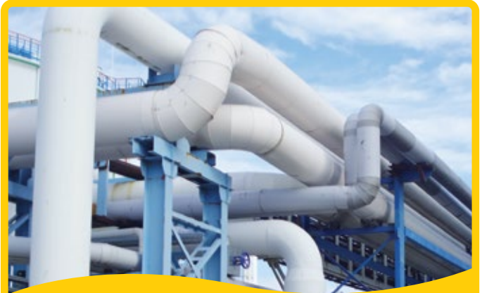
ASSEMBLY OF PIPE SPOOLS
