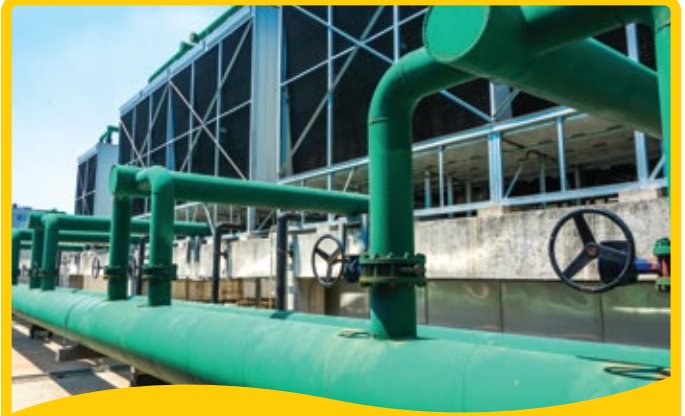
WATER TREATMENT – OPERATION & MAINTENANCE OF RO, STP PLANTS
