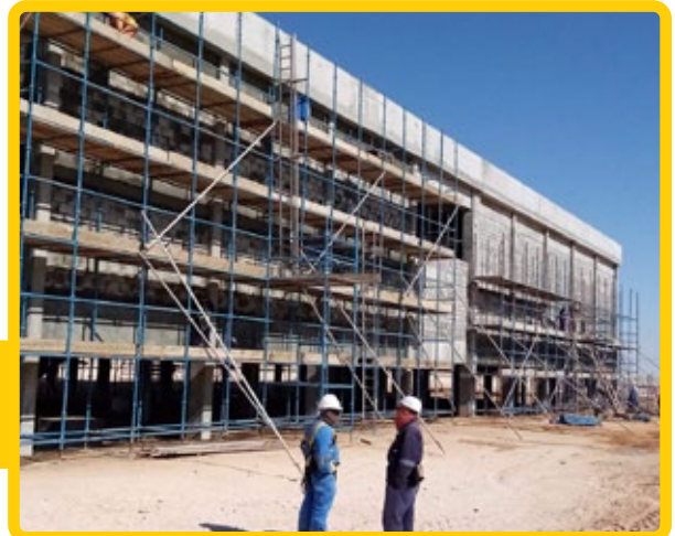
9. CONSTRUCTION OF CONTROL STATION BUILDING FOR AIP PDO AT BIRBA
