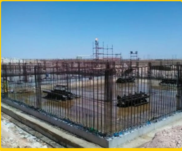
16. CONSTRUCTION OF CHEMICAL TANK FOR STS PDO AT AMAL
