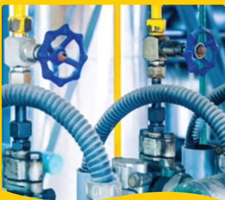
REPAIR & MAINTENANCE - VALVES & PUMPS
