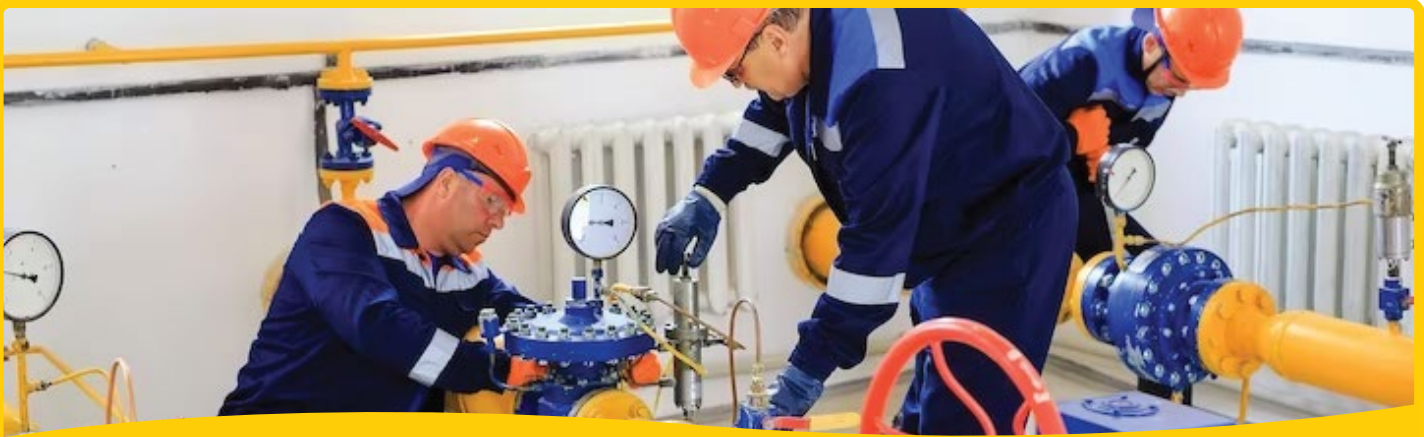
HYDRO TESTING OF PIPES
