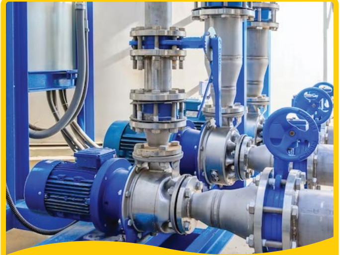
DEMOLITION OF REDUNDANT PIPELINE, PUMP, MOTORS, MSVS, EQUIPMENT ETC.
