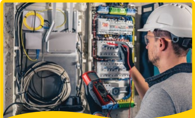
INSTRUMENTATION – PLC & SCADA SUPPORT
