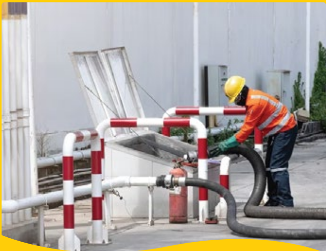
DRAINING AND FLUSHING OF PIPELINES
