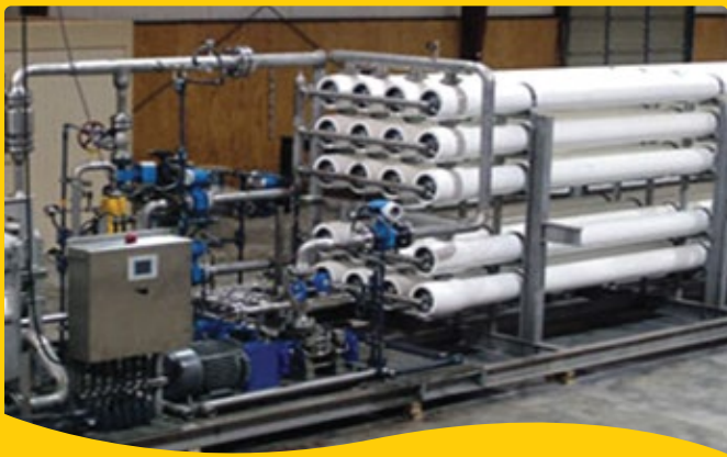
WATER TREATMENT – SUPPLY INSTALLATION AND COMMISSIONING
