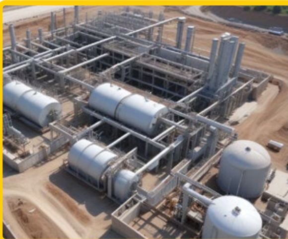
5. CONSTRUCTION OF STP PLANT CIVIL & MECHANICAL
