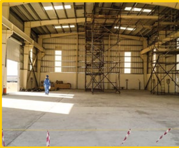
13. CONSTRUCTION OF FABRICATION SHOP FOR AIP PDO AT AMAL
