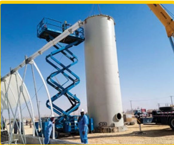
15. CONSTRUCTION OF MECHANICAL WORK FOR AIP PDO AT AMAL
