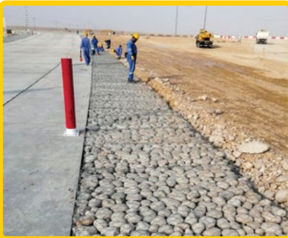
10. CONSTRUCTION OF GABION RIPRAP WORK FOR AIP PDO AT AMAL
