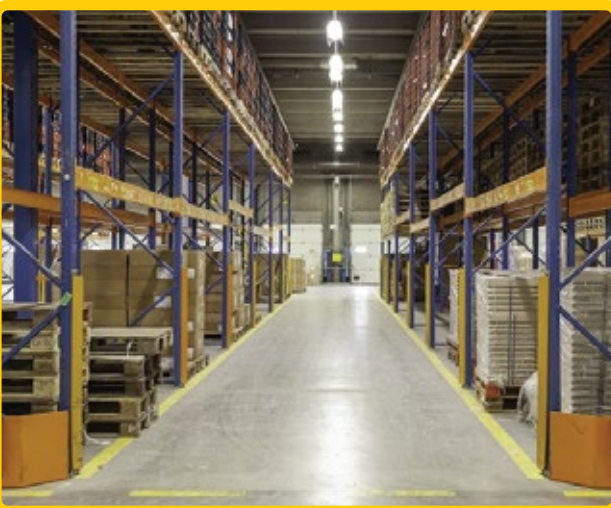
3. FABRICATE & ERECTION OF WARE HOUSES
